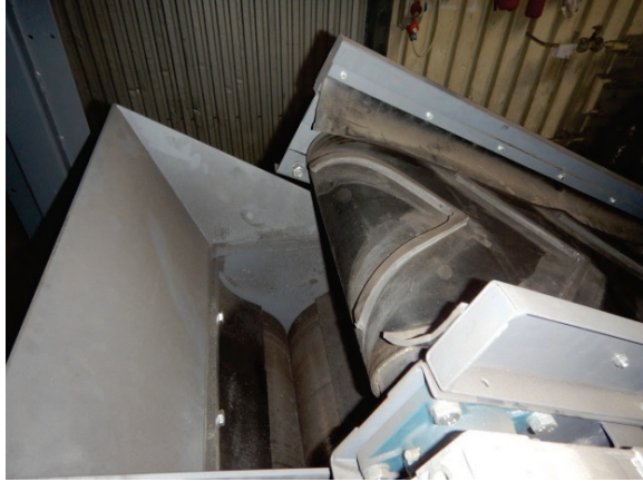
Fig. 11. Access to the rollers of the crusher
