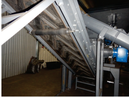
Fig. 5. The places of catching under the conveyor (between the belt and rollers and between the belt and the frame)
